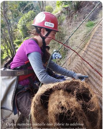
Corps member installs coir fabric to address erosion control after removing invasive plants from a hillside.
