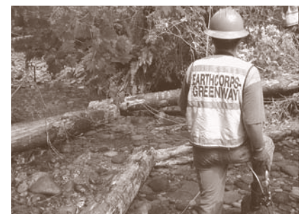
EarthCorps installs large woody debris to make streams more hospitable to salmon and other wildlife.
