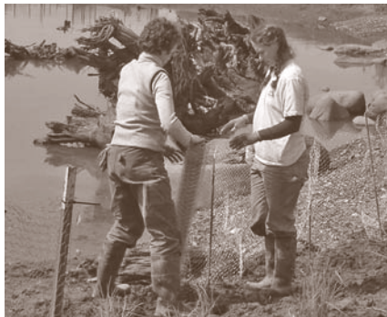
Corps members Jill Politsch and Megan Hess install the frame for a goose exclusion system in Mowitch in Tacoma's Commencement Bay.
